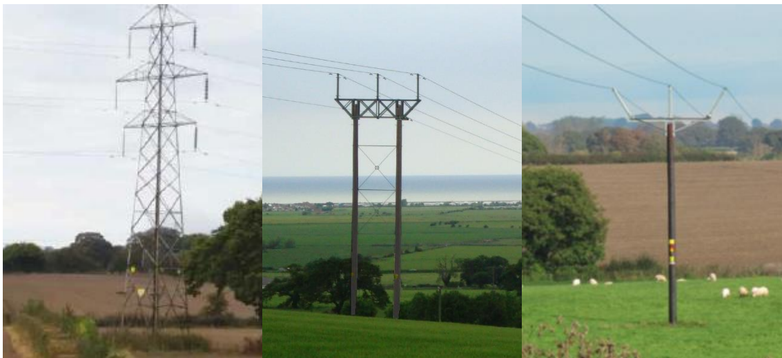
Steel pylons – approx. 26m Heavy duty double wood poles – approx. 15m Single wood pole Trident – approx. 12m
